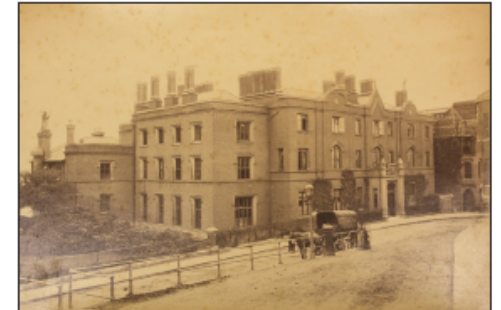
View of The Head Master's Boarding House (late C19)
